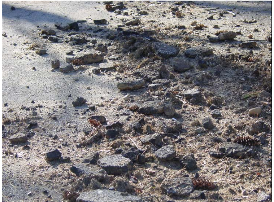
April 21, 2007 - For the past several years we have had to clean up broken asphalt each spring after the snow banks melt. Pictured above is only a small portion of this year's deposit.
